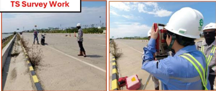
TS Survey Work
